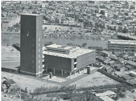
The facade of Fukuoka Prefectural Culture Center c.1964: Photo by unknown
